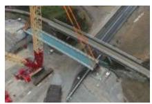
The new bridge weighs 275 tonnes, the equivalent weight of 23 double decker buses or 887,097 standard Cornish pasties and will eventually span the existing A30 road and four lanes of the new carriageway. Now in position, work will concentrate on construction of the new road, with the existing bridge to be demolished later this year.
